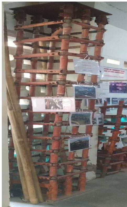
Figure 2.2 Batteded column (Chauhan, 2012)
