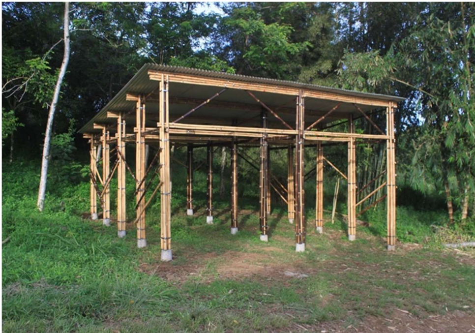
Figure 5.4 Lightly loaded temporary bamboo
