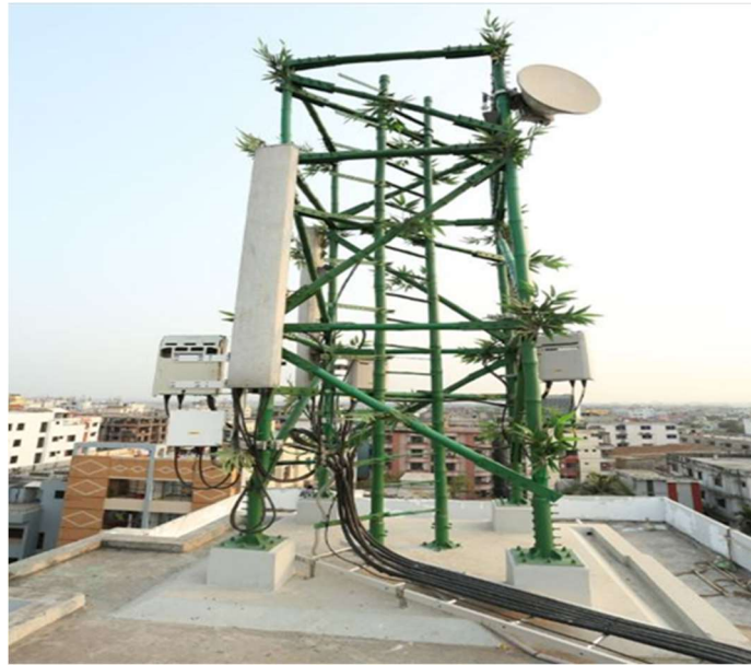
Figure 5.3 Light batted bamboo structure for light load
