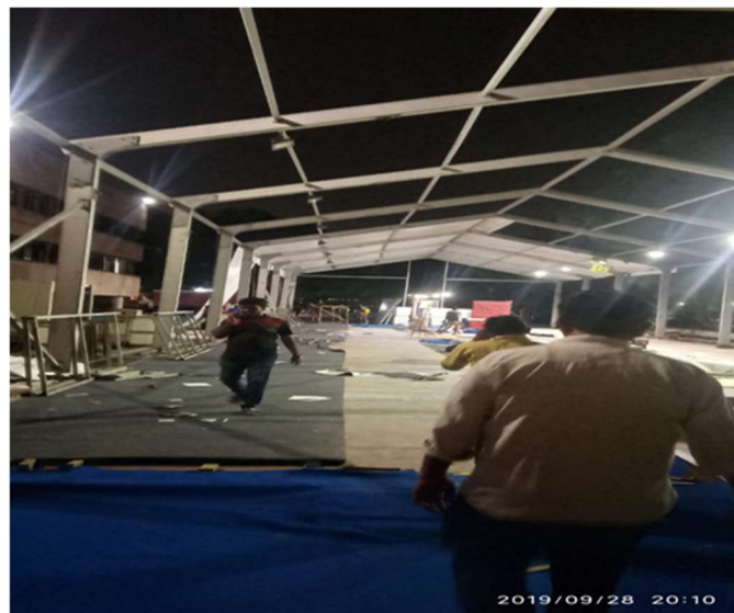
Figure 5.6 Temporary steel shed in IITD
