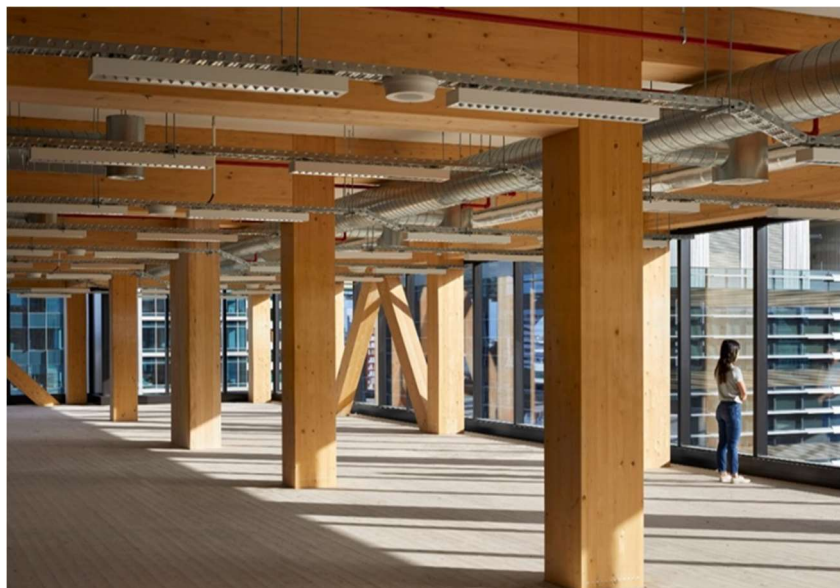
Figure 5.2 Timber beam and column used in timber building
